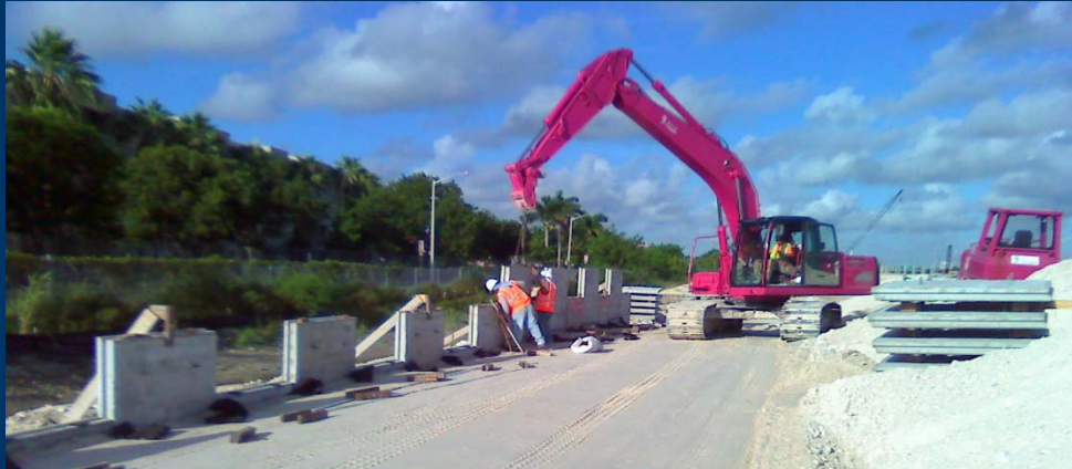
Crews construct a retained earth wall south of S.R. 836
